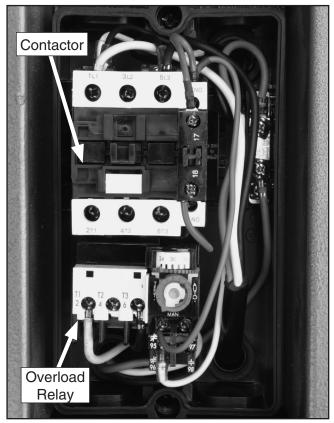
Figure 87. G0591 single phase magnetic switch.
